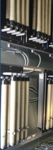
**AtmosAir Model 508FCs rack-mounted systems in an AHU.**
